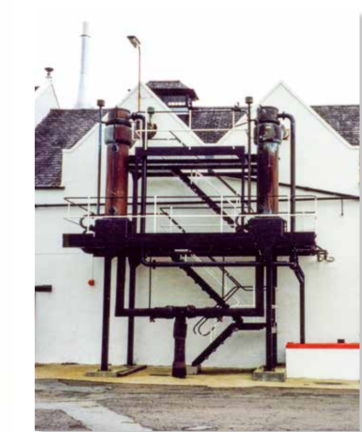
For seven years, the distillery used shell and tub condensers
